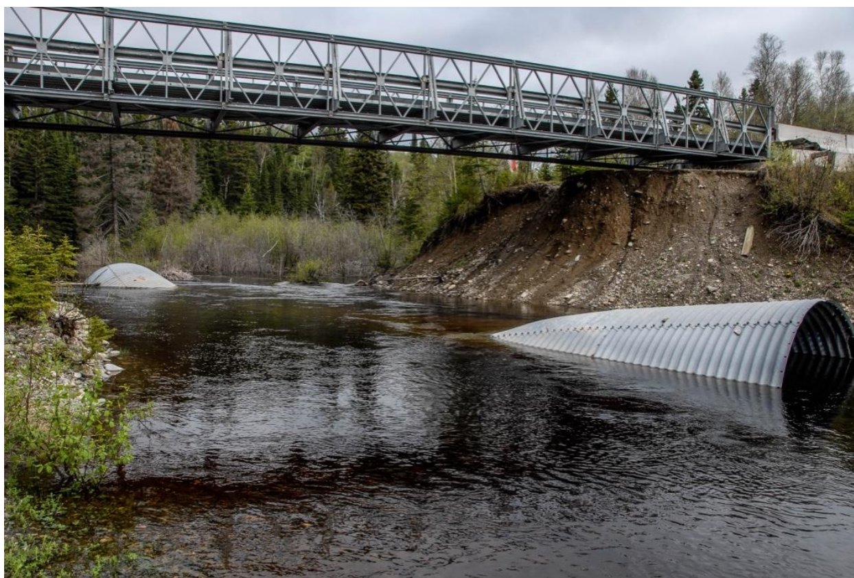
Washed-out culvert and temporary bridge installation in Wawa. Photovoice participant 6 (2016)
