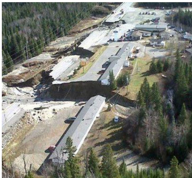
A section of washed-out trans-Canada highway 17 and damaged motel from the 2012 flood in Wawa, Ontario. CBC
